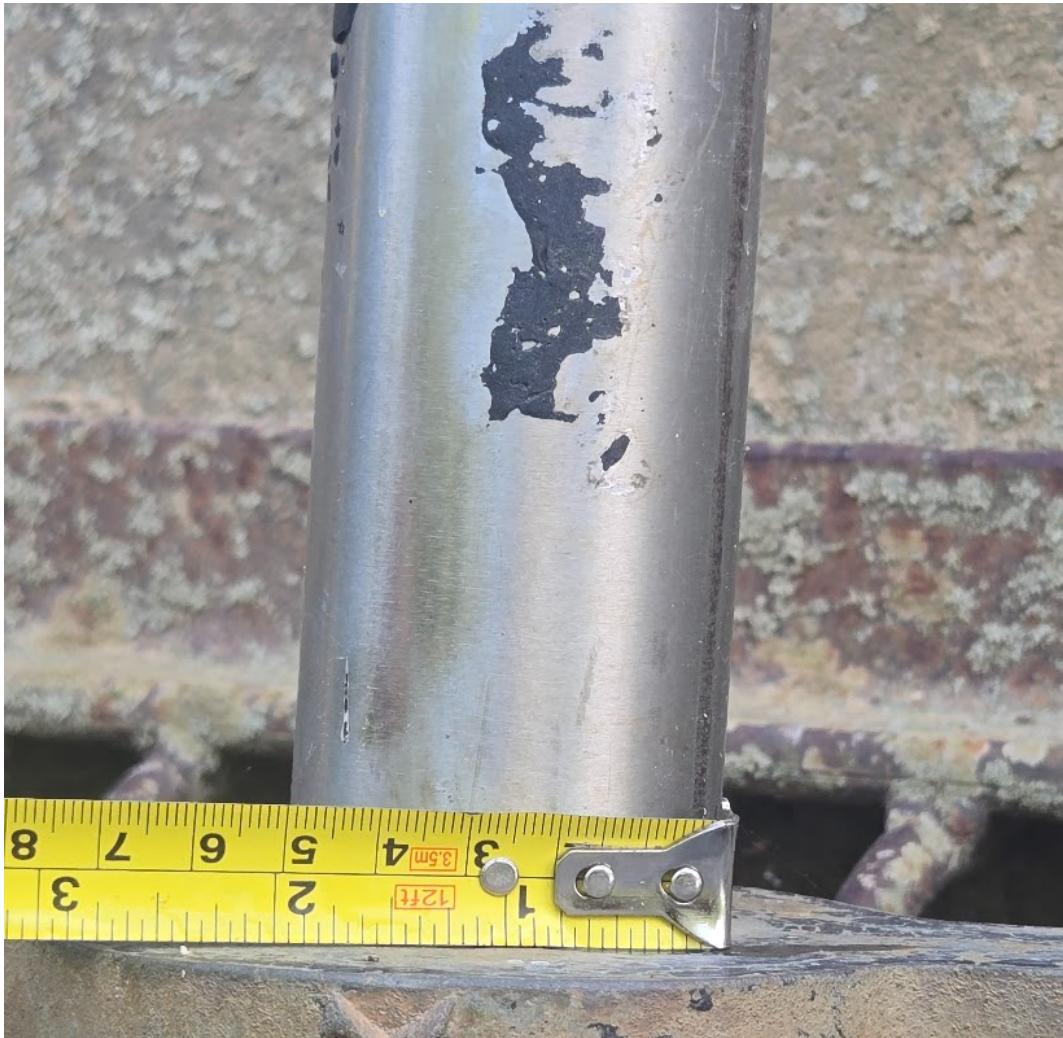
Existing Sluice Gate stem and mounting
