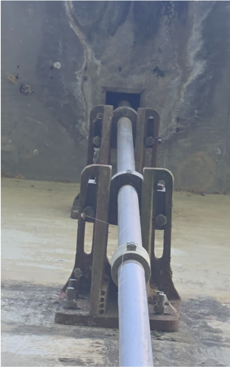
Existing Sluice Gate stem
