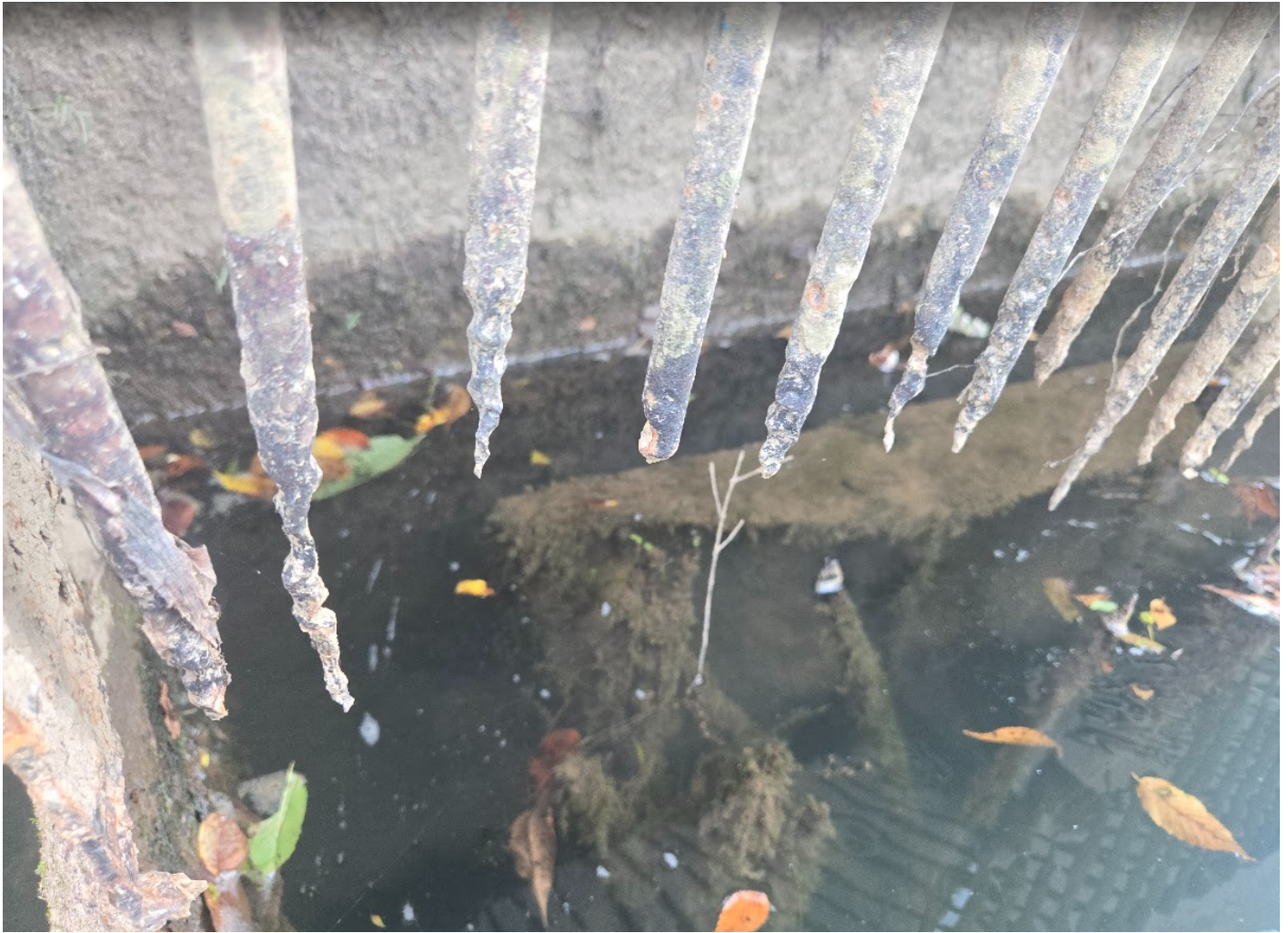
Exterior Sluice Gate and Bar Screen
