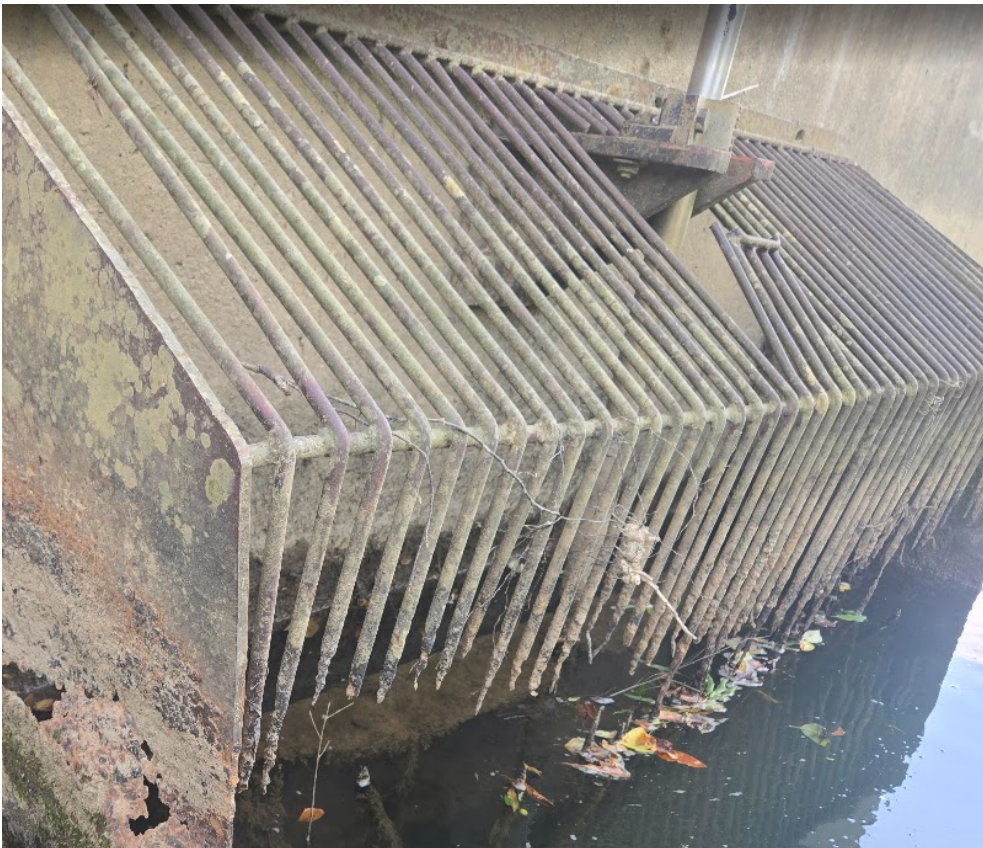
Exterior Sluice Gate and Bar Screen
