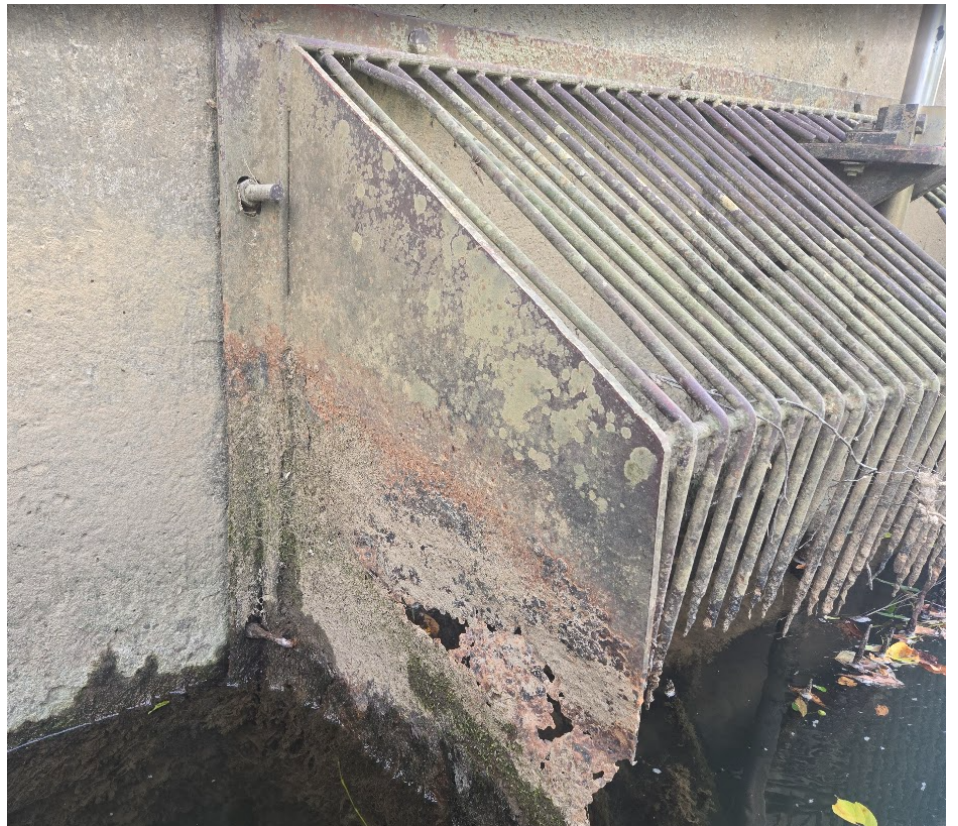
Existing Sluice Gate stem and mounting
